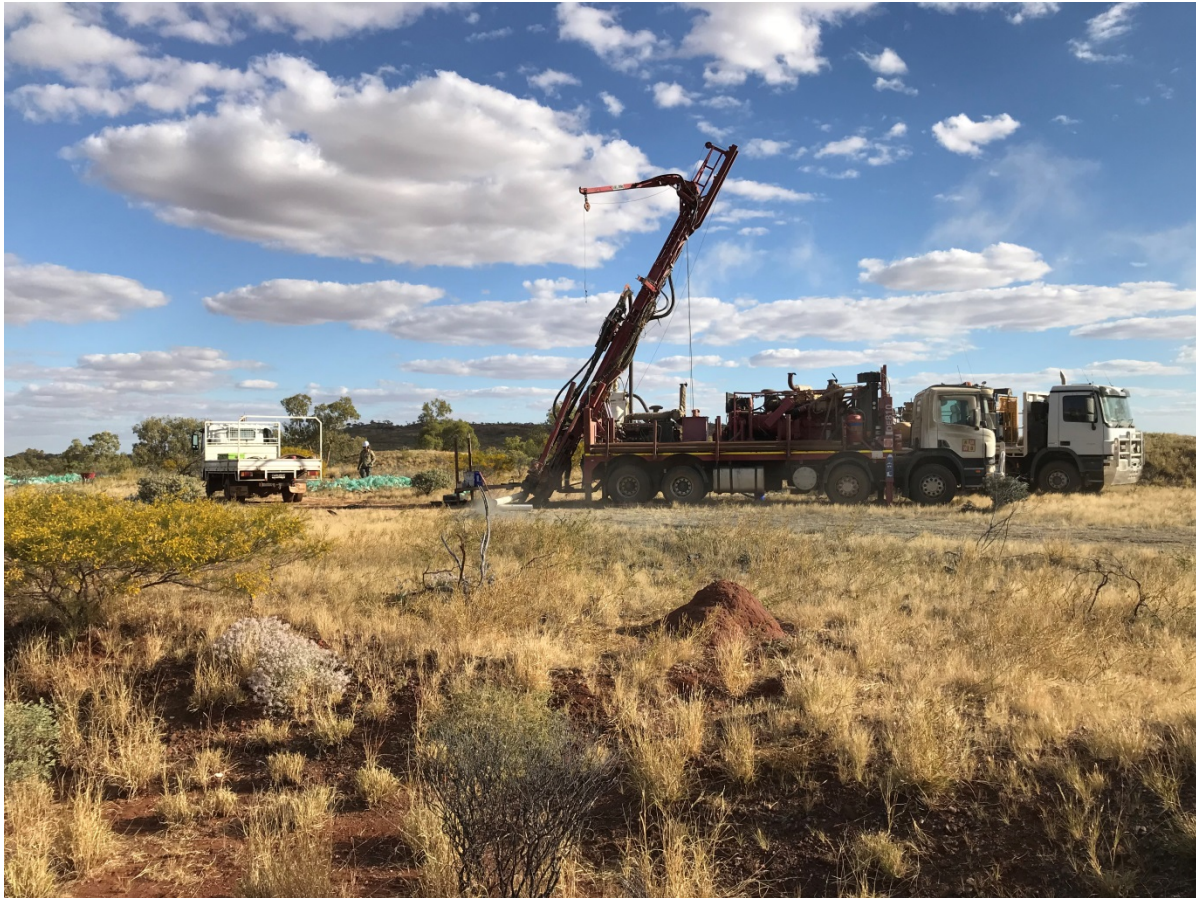
Figure 2: Reverse circulation drilling underway at Mount Birnie.
