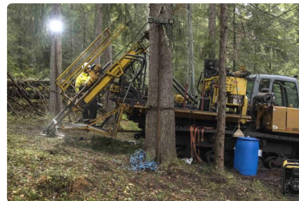
Drilling at Middagshville
