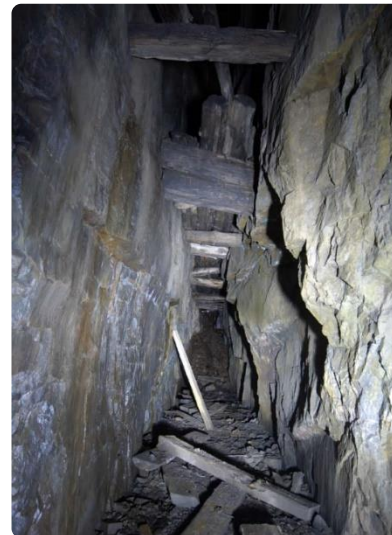
Gladhammar historic cobalt workings (source: Gunnvall, Gunvall and Aren, 2008)
